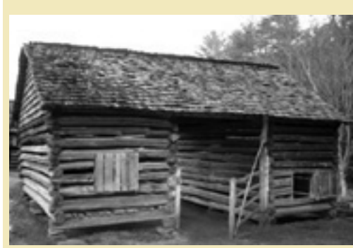
Typical double-pen corn crib, Pickens County, South Carolina
