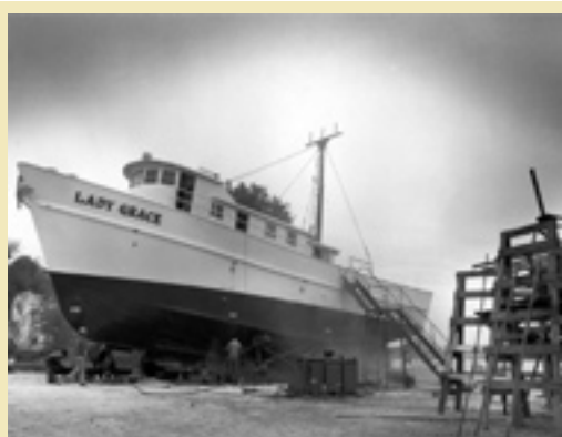
Trawler Lady Grace. Second steel trawler built by Beaufort Industrial Marine Company Inc., Lady's Island, 1969.
